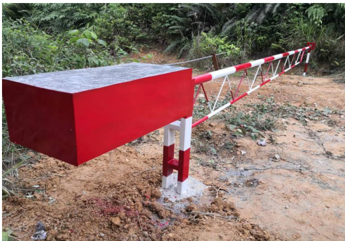
New Gate Installation
